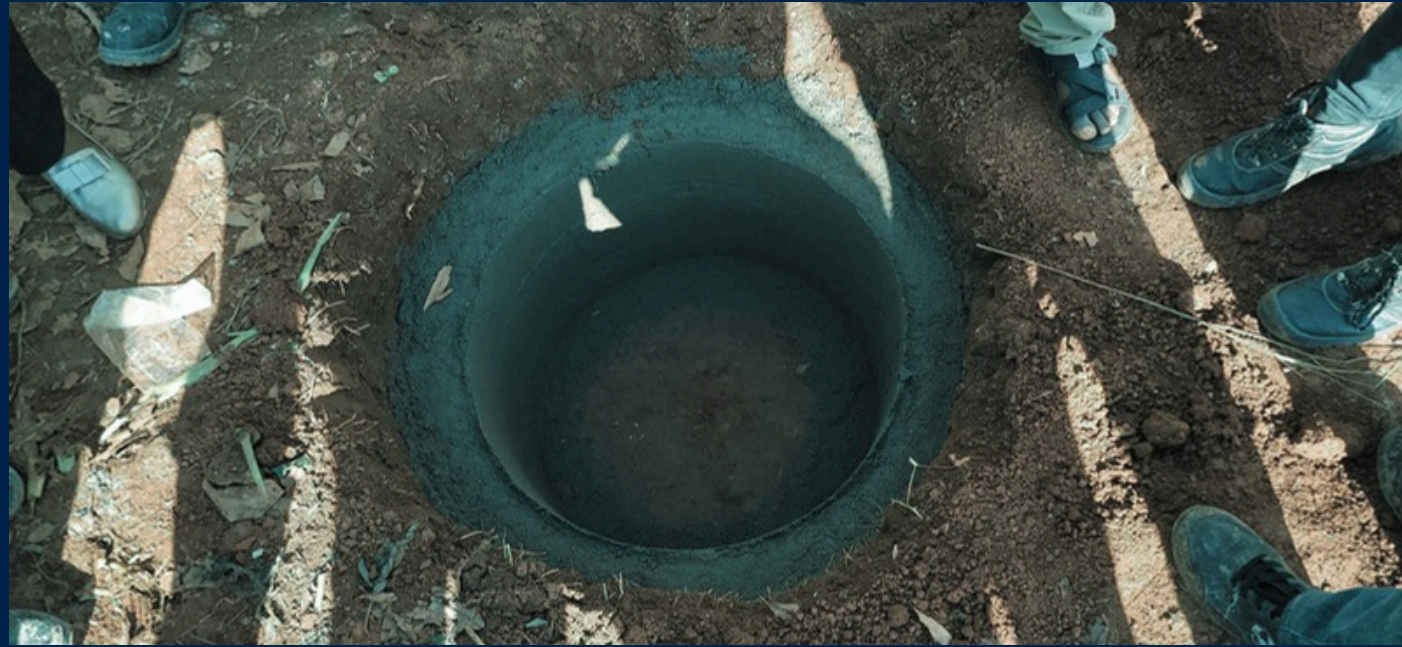
constructed pit lining
